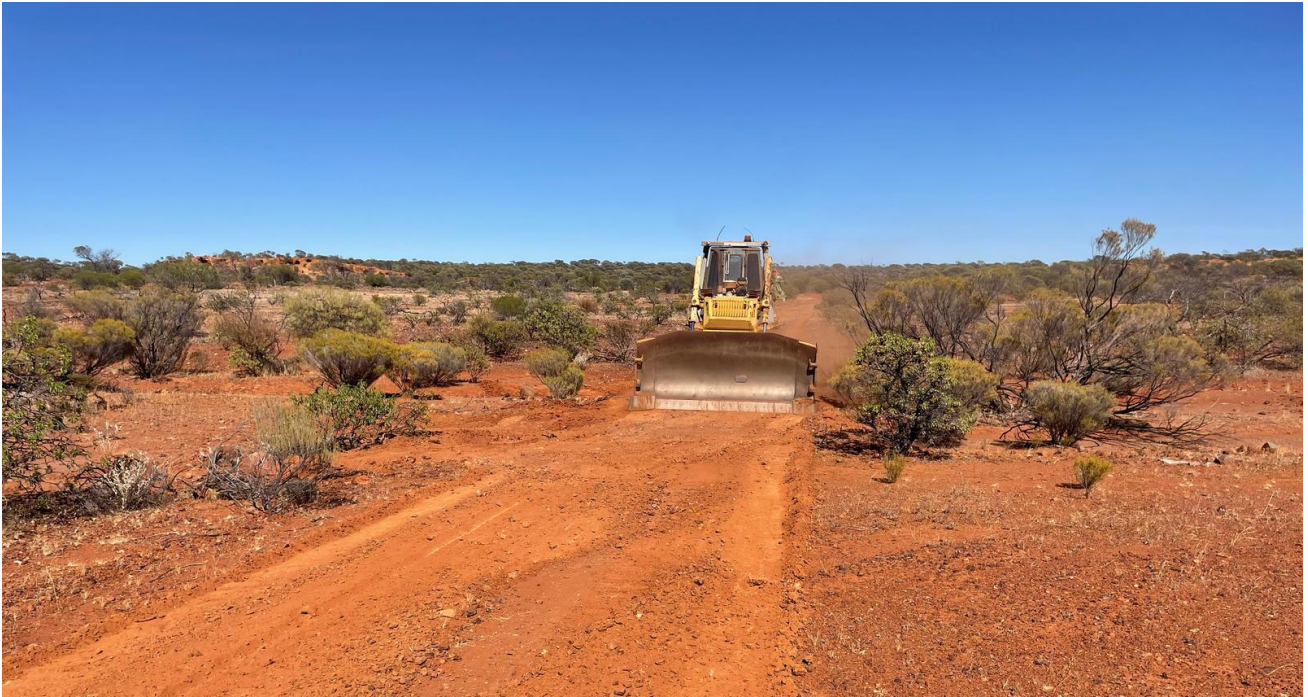
Figure 1: Site works commencing for March drilling program
