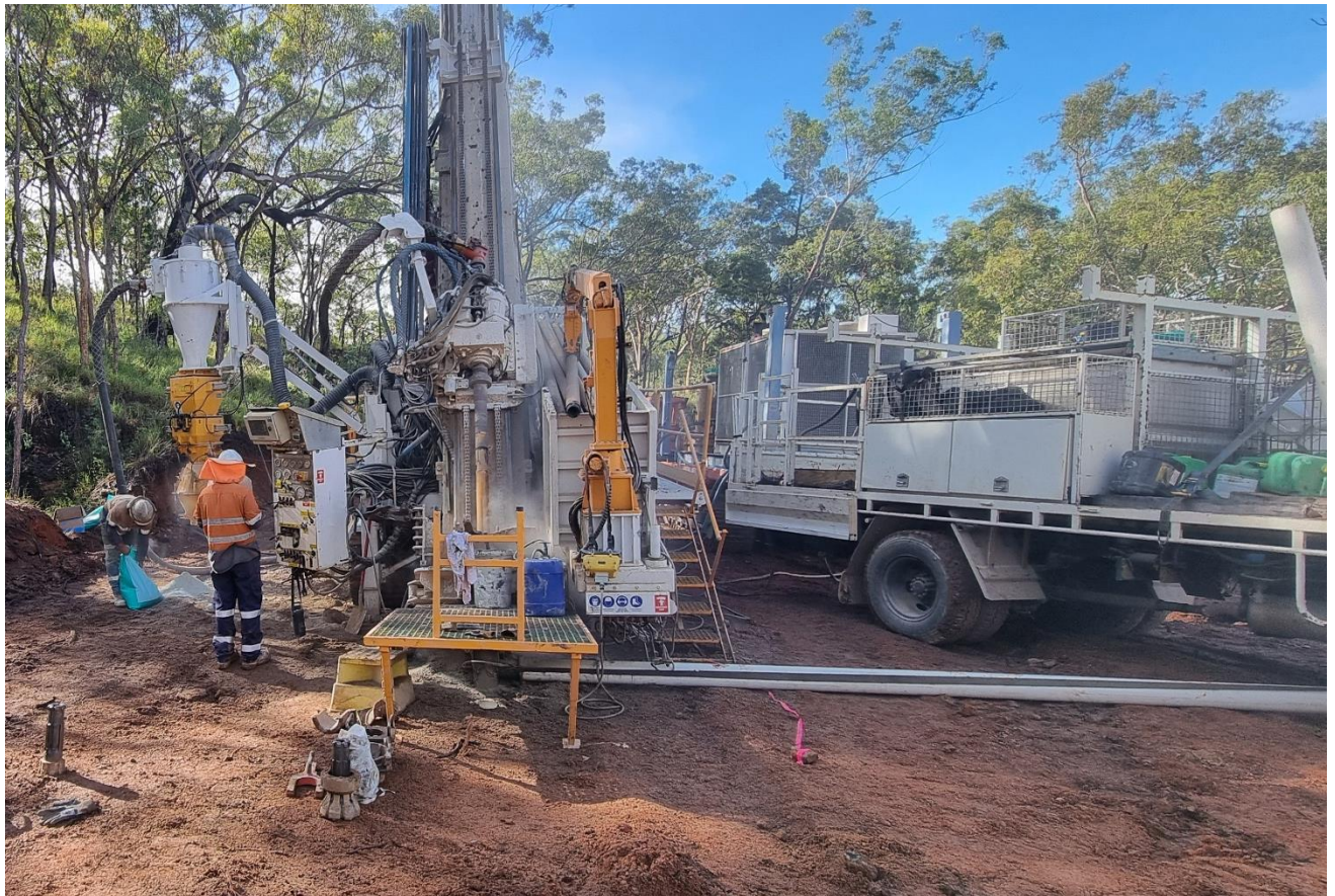
Figure 2 Track-mounted reverse circulation (RC) drill rig at Orient West (ORR070)
