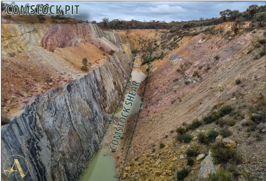
Figure 2: View to Southwest of Comstock Open Pit Showing Target Comstock Shear Zone.
