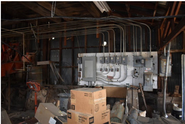
Photo 3. Electrical control board within the mill building.
