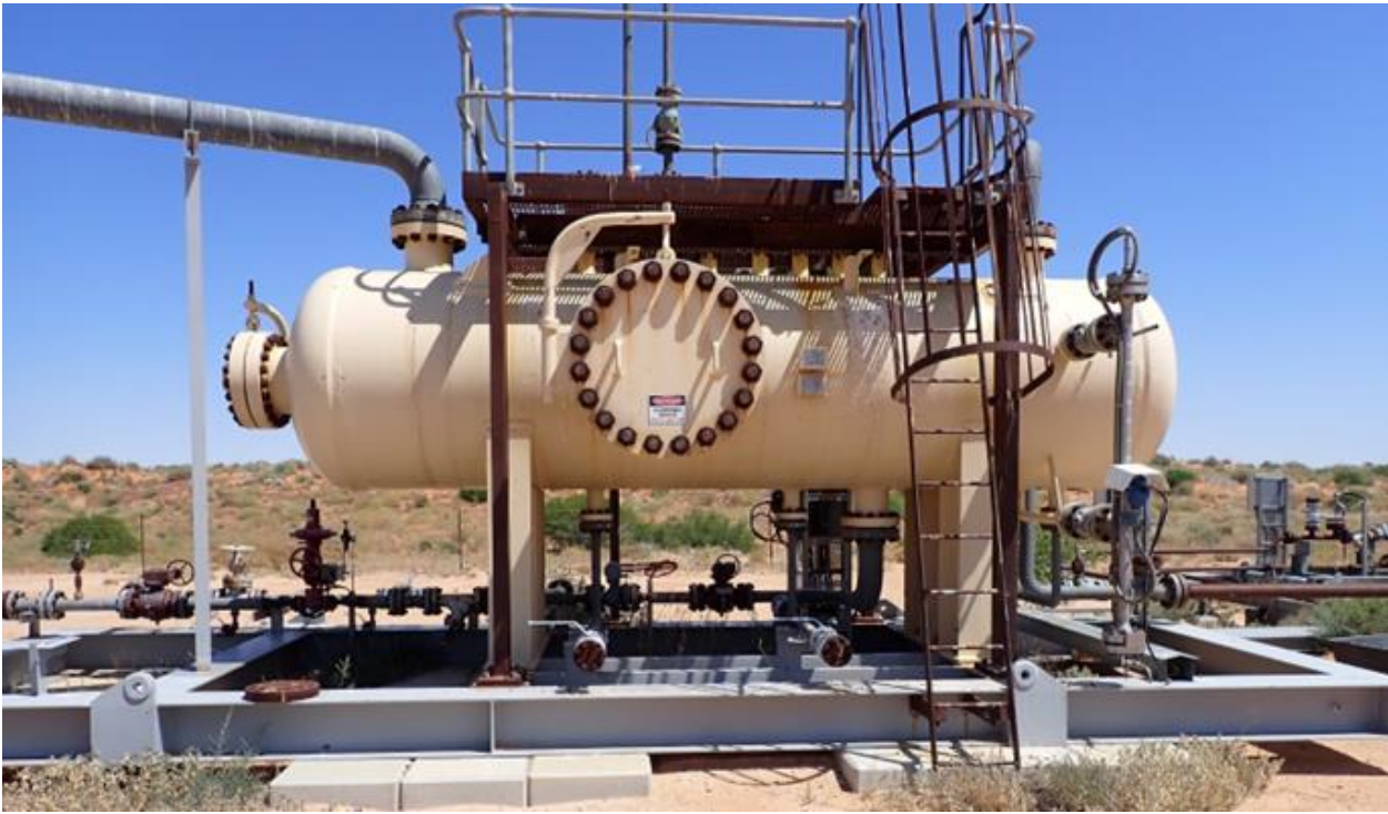
Figure 3: Gas/liquids separator in place at Vanessa facility.
