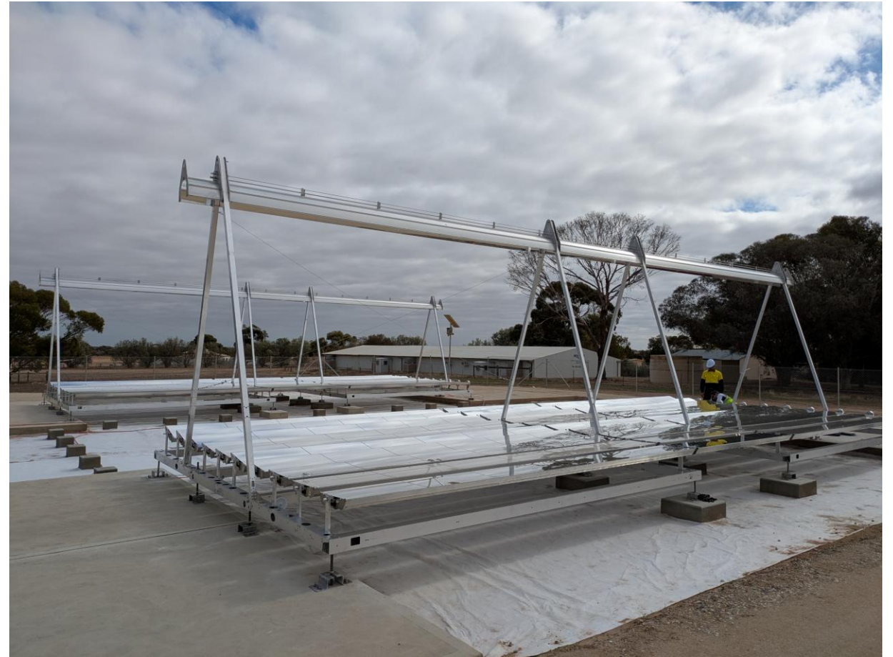
LFR Installation at the Roseworthy pilot plant during mid May 2025
