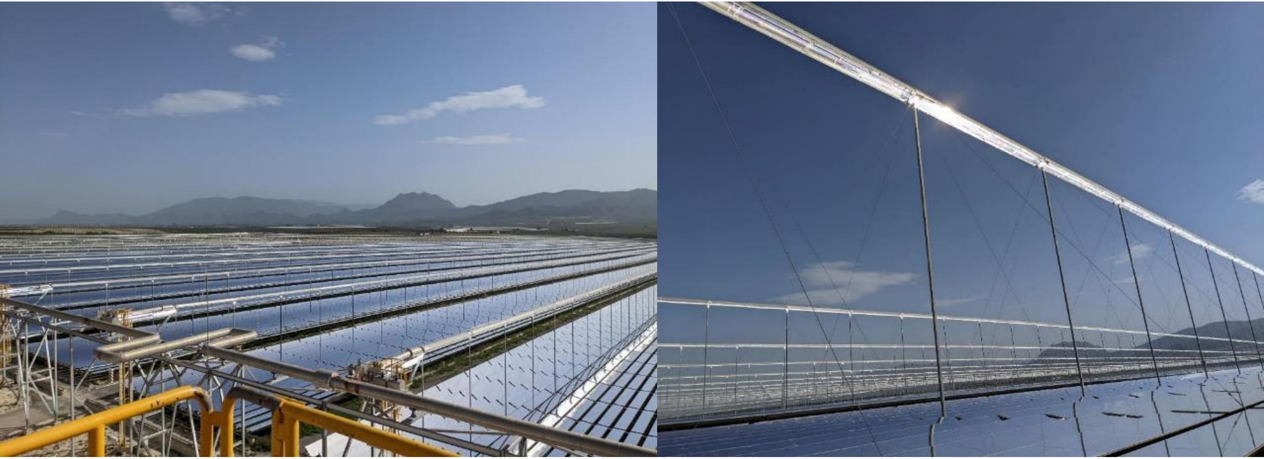
Commercial scale linear Fresnel field in Spain (28 x ~1km mirror rows) generating ~30MW electricity
