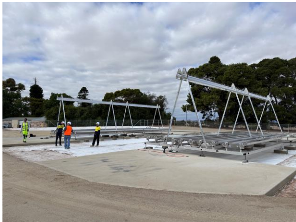
LFR erection at site
