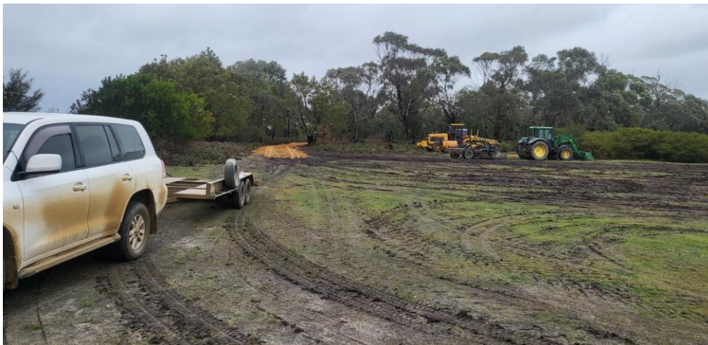
Figure 1: Early stage of Wombat-5 Site Works
