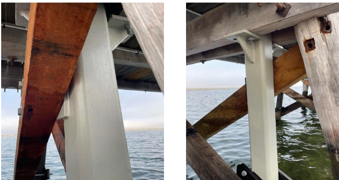
Figure 2: Trial inspection photos showing coatings performing well at the Streaky Bay Jetty, South Australia (April 2025)
