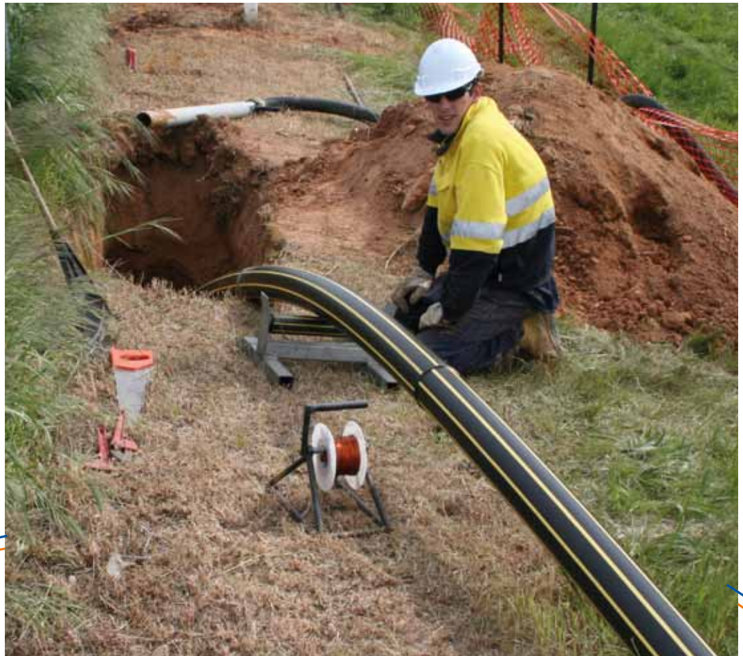
Laying gas pipe using the direct drilling method reduces the disruption caused by open trenching.
