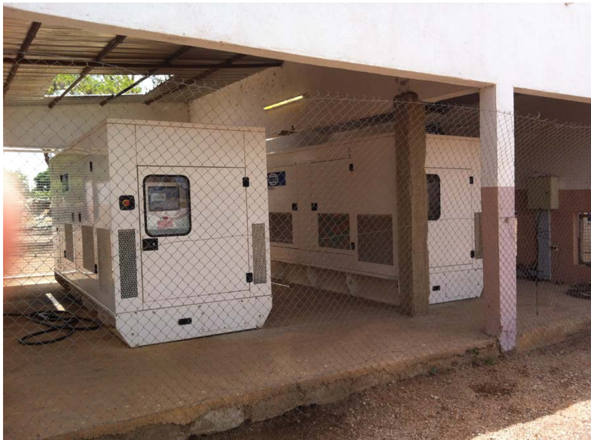
Figure 20 - Two Wilson gensets (1 duty, 1 standby) providing power to the Douta Camp.
