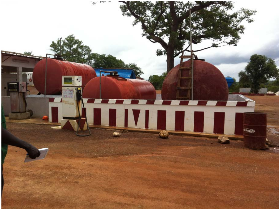
Figure 19 – 85,000 litre diesel fuel farm within the Douta Camp.
