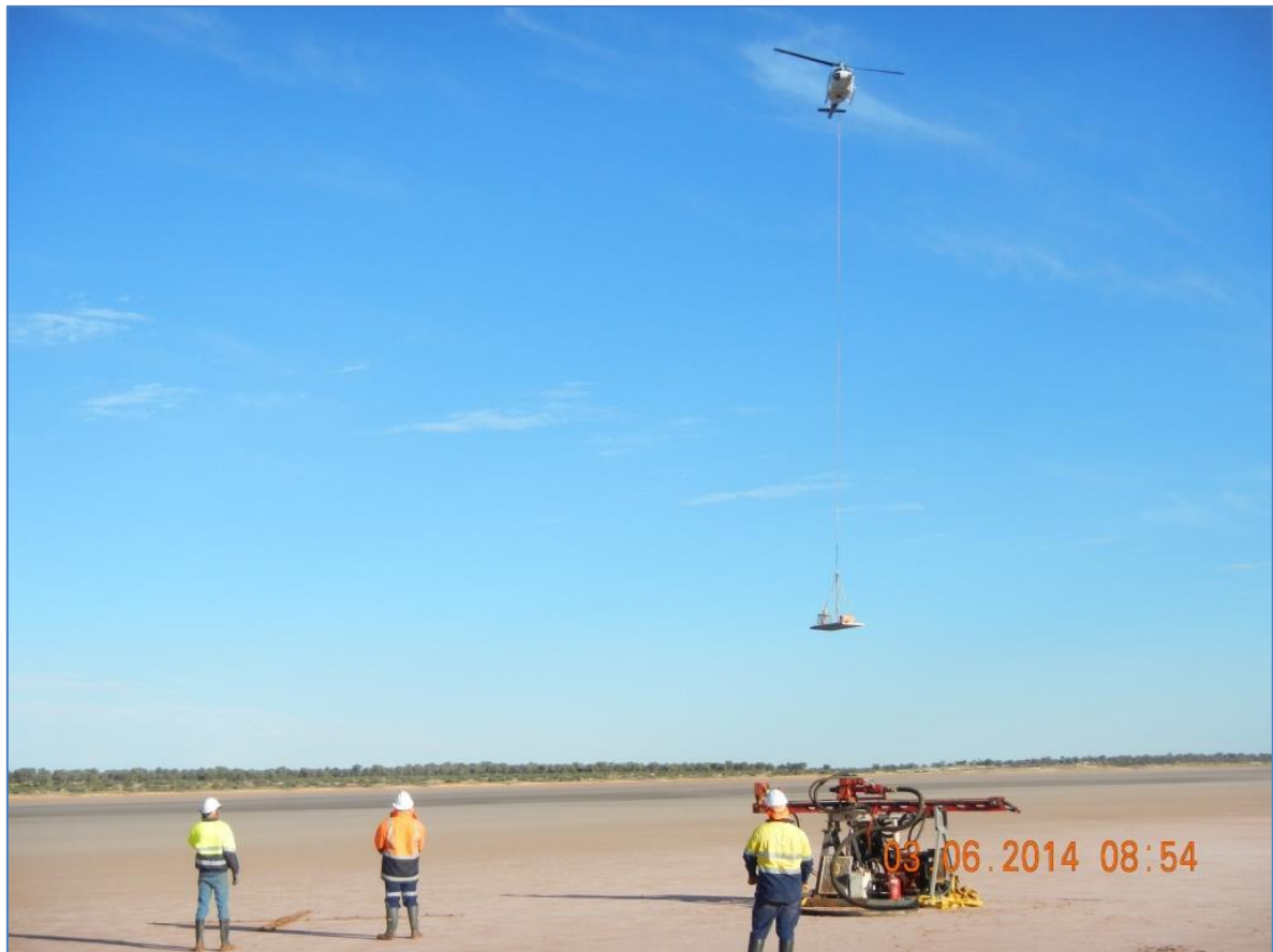
Figure 4. Support pontoon being lowered into position by the helicopter.
