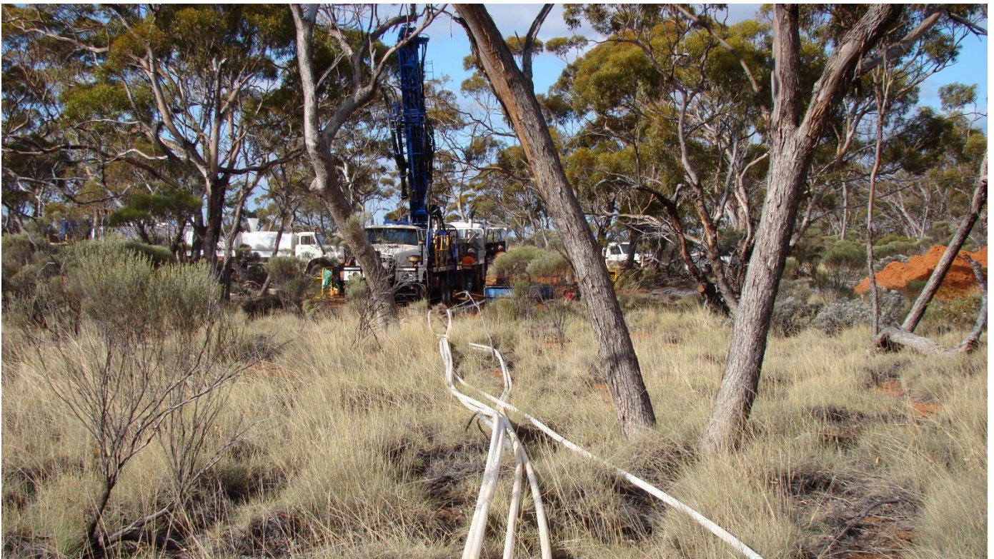
Photo 7. PVC laid out on ground ahead of running down the hole for down hole electromagnetic survey
