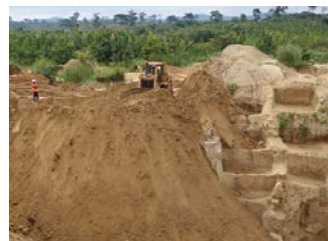
Filling in artisanal workings at Hiré
