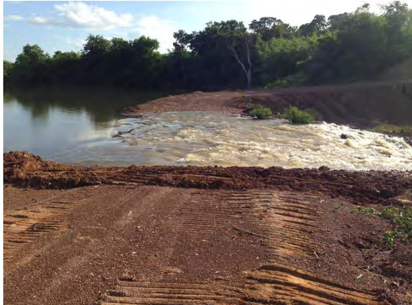
**Figure 8 – Water Storage Dam Spillway**
