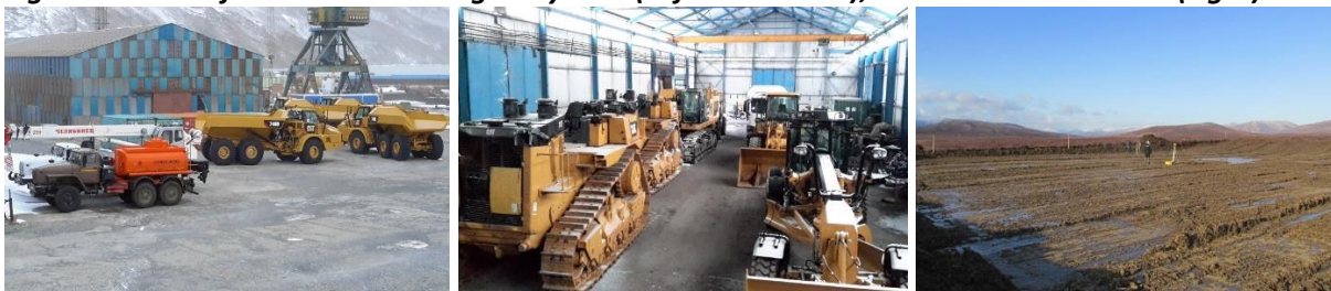
Figure 17: Mine fleet at TIG’s Beringovsky Port (Left and Centre), Fuel Farm Earthworks (right)
