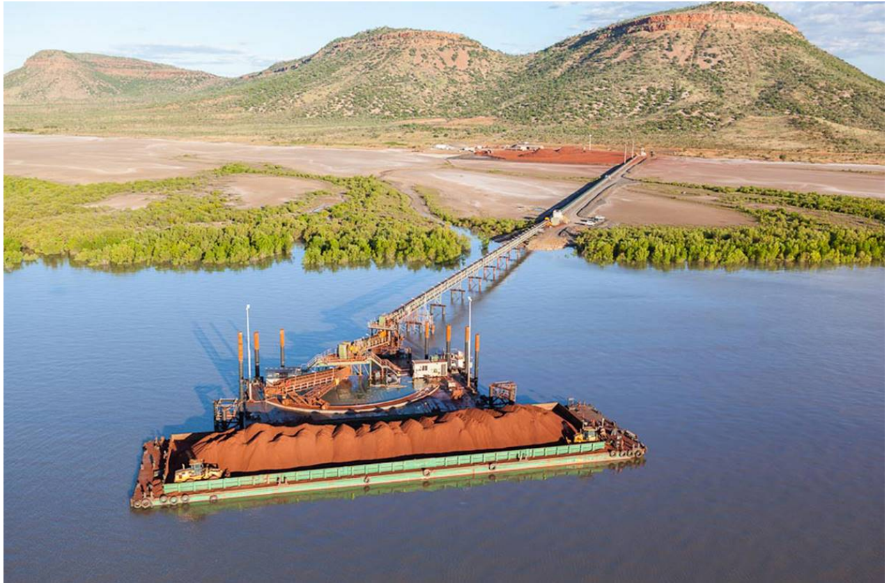
Figure 4 | Aerial view of an 'A' Frame jetty with ore loading onto a waiting barge or TSV
