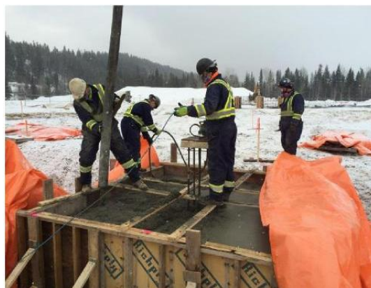
Figures 3 & 4 Concrete pouring at Moberly Plant site
