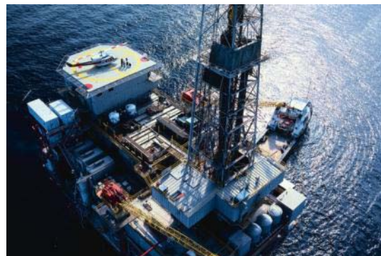
Shallow Water Drilling
