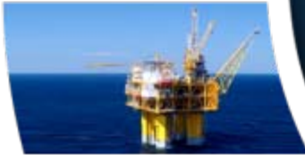
Oil & Gas Platforms & OSVs
