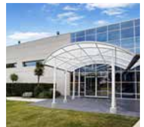
GE BUILDINGS 1&3, 572-576 SWAN ST, RICHMOND, VIC
