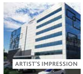
211 WELLINGTON RD, MULGRAVE, VIC (to be constructed)
