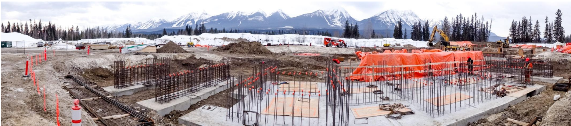
Moberly Plant Site –footings for silos
