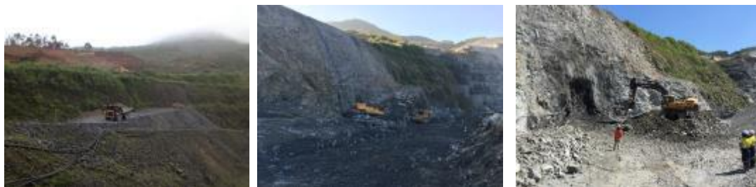
Bacbacan Ramp Earthworks
