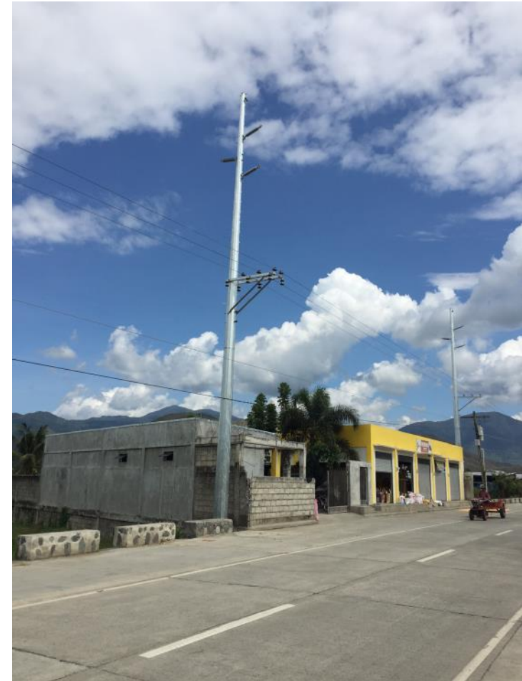
Stage 1 pole installation progress
