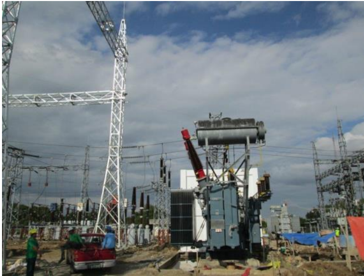
Stage 2 NGCP Substation Transformer installation at Bayombong in progress
