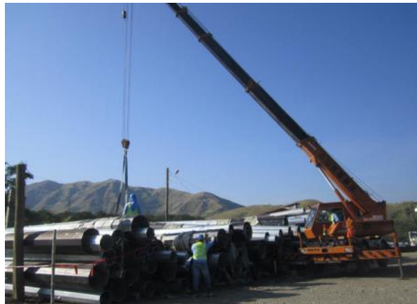
Stage 1 pole staging
