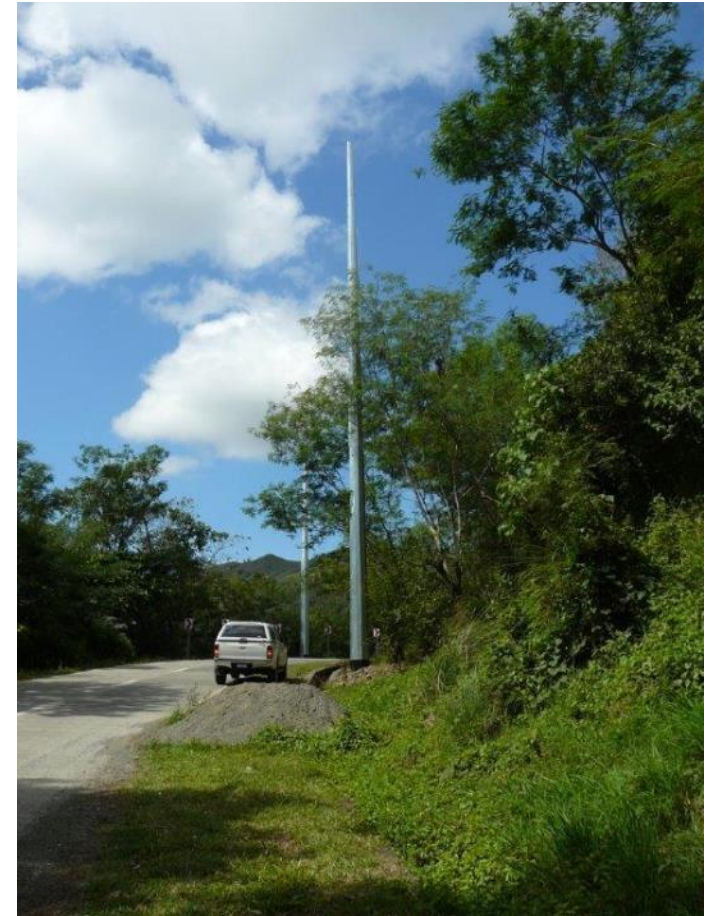
Stage 1 pole installation progress
