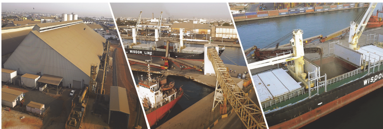
Storage and conveyor facilities at Dakar Port
