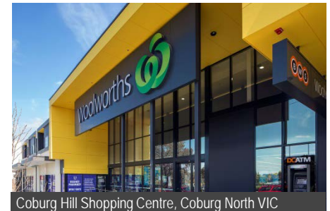
Coburg Hill Shopping Centre, Coburg North VIC
