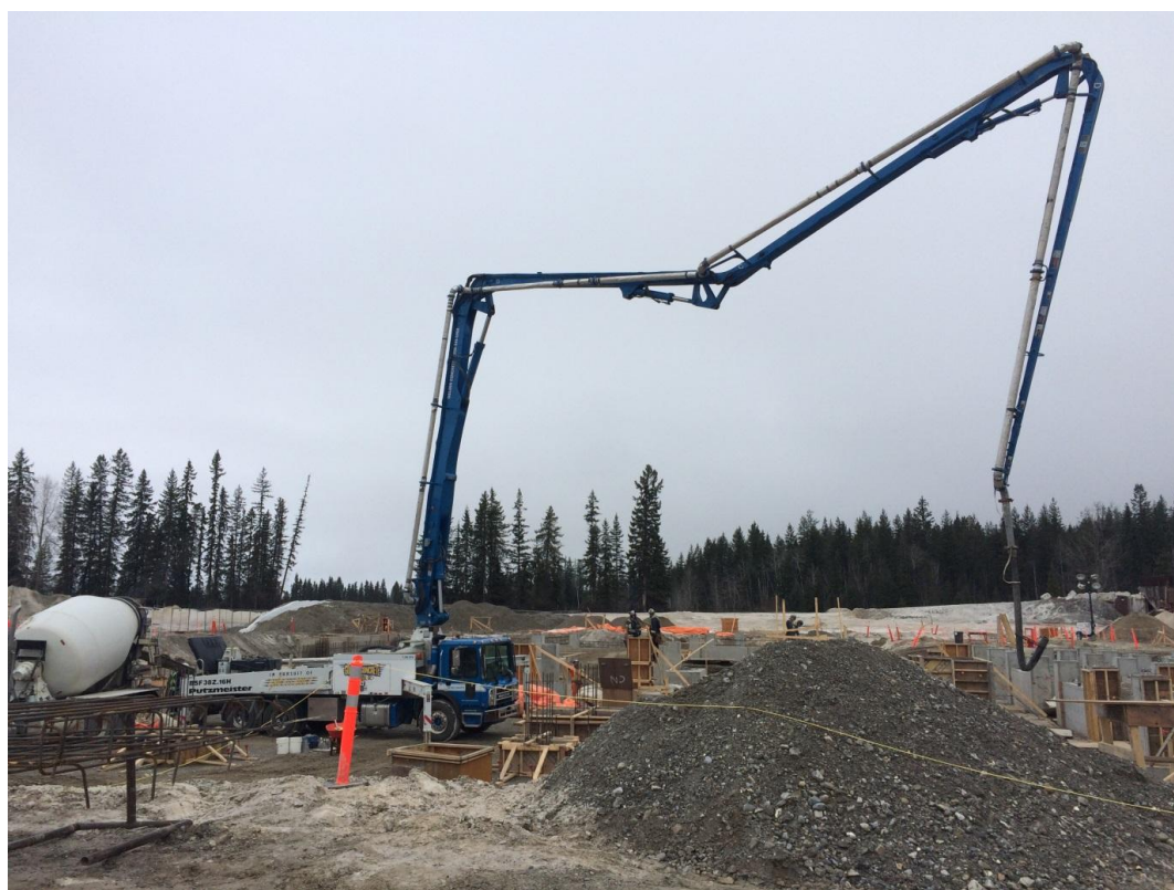
Figure 2 Moberly Plant Site – concrete pour work on the main process building
