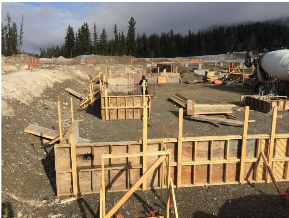
Figure 3 Process building framework under construction
