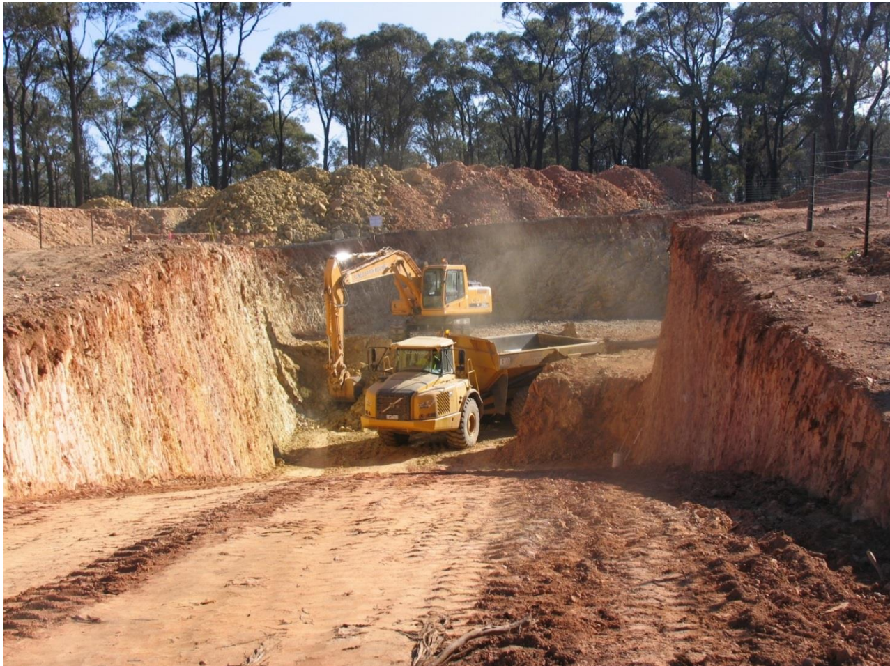
Figure 4: Test pit looking West
