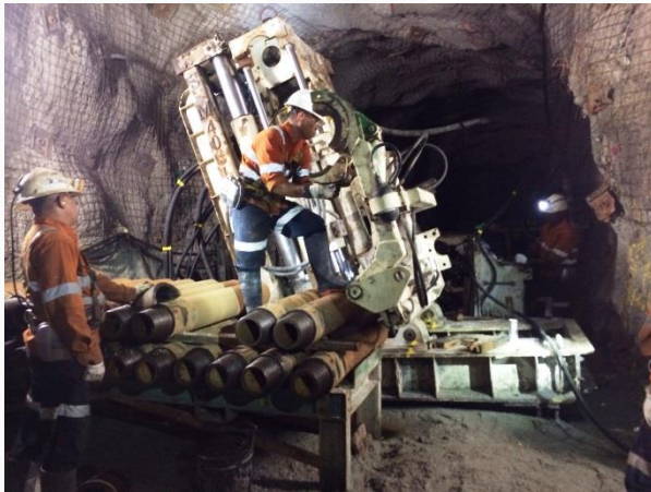
Bore hole machine in operation
