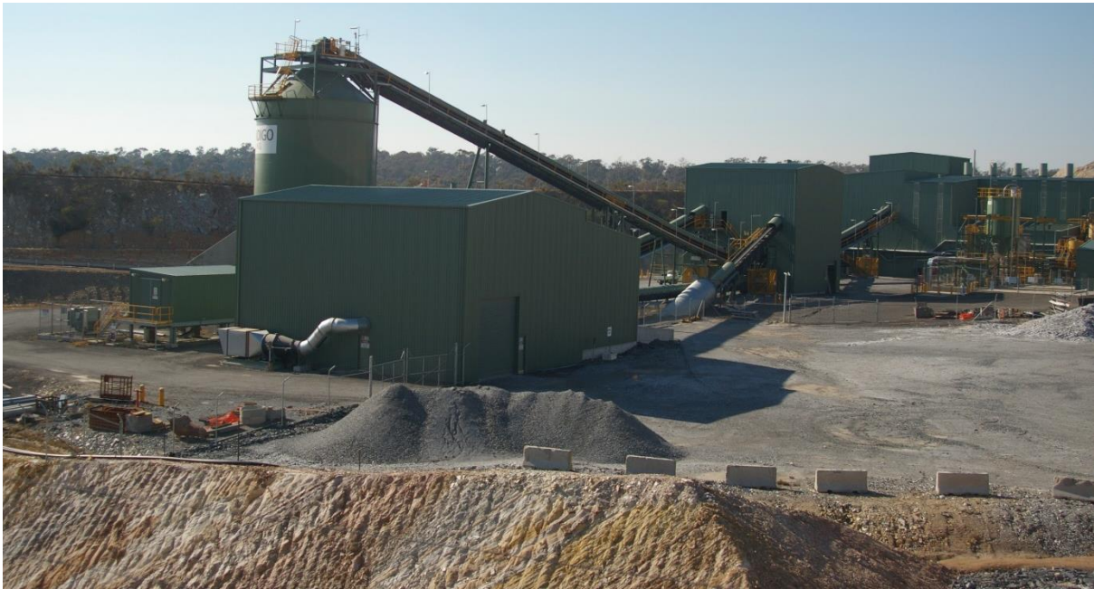
Figure 4: Kangaroo Flat 600,000tpa Gold Processing Plant
