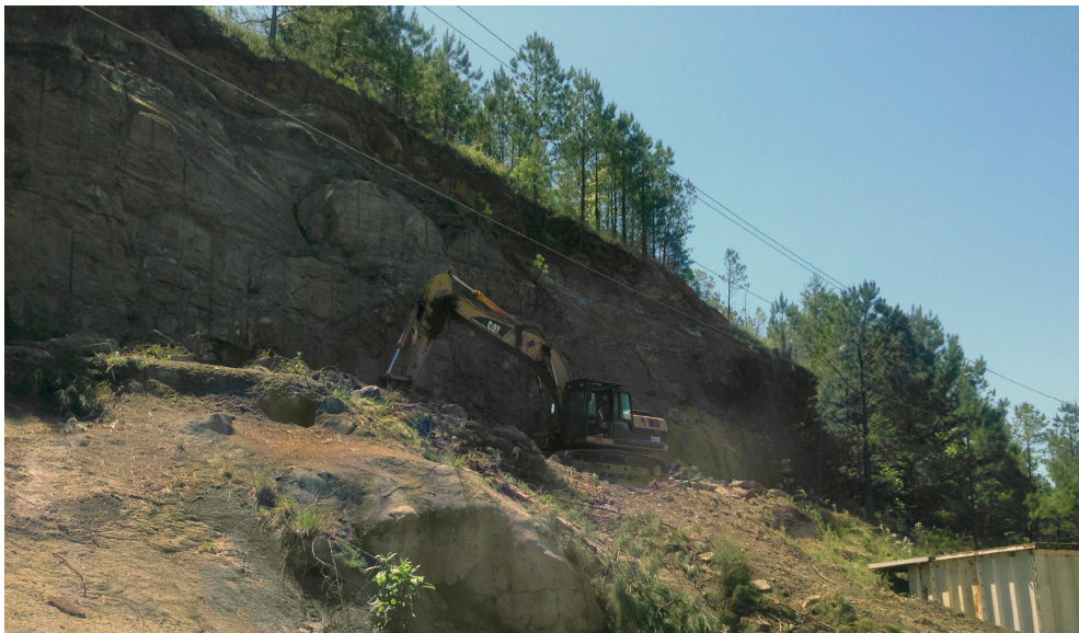
Figure 2: Highwall preparation in readiness for mine re-entry
