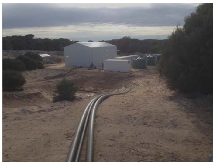
Perth Wave Energy Project pipelines connected to the power house and desalination plant, Garden Island, WA
