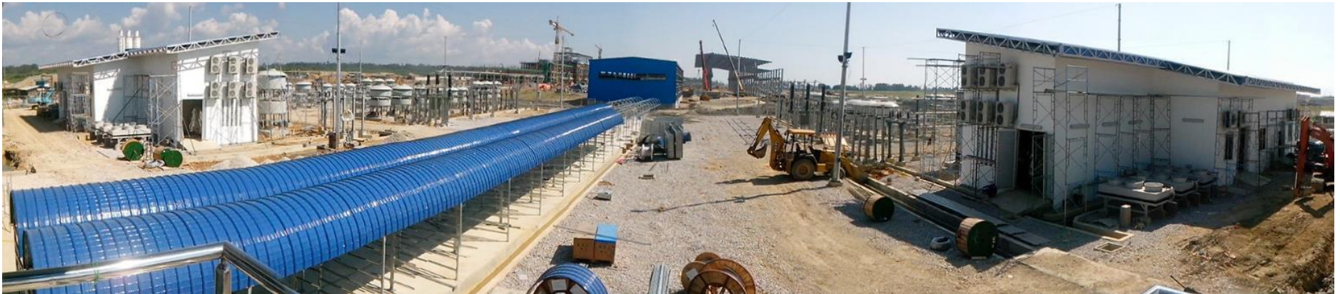
SVC yard, capacitors, control building, and cable tray from 275 kV Substation to the Smelting Plant
