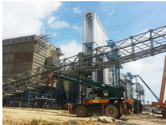
A1 Deduster and feedstock conveyor
