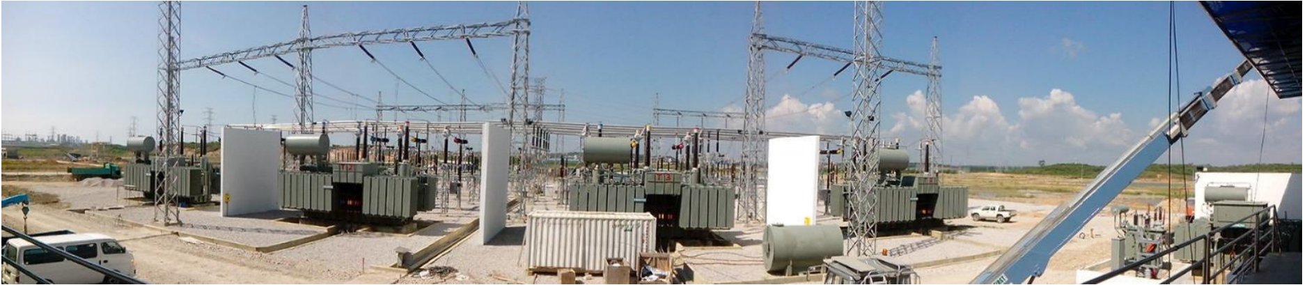
Incoming line from SESCO and 4 x 180 MVA transformers
