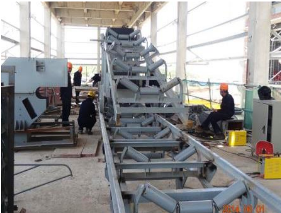
Belt Conveyor installation
