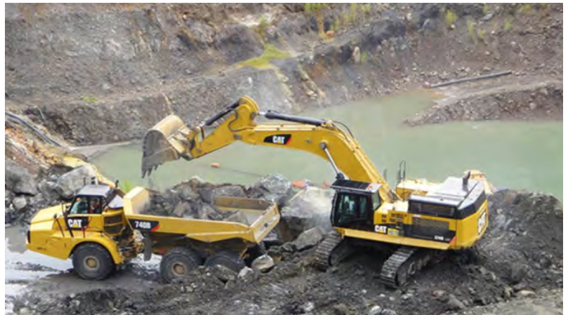
Durable rock fill, being loaded for TSF3 construction.
