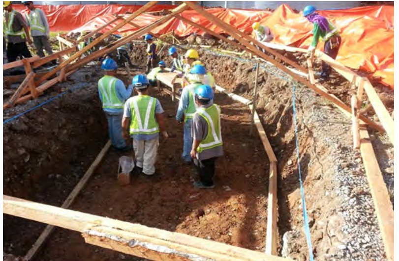
Foundations for the thickener plant.
