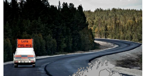
Road through Nunasvaara project
