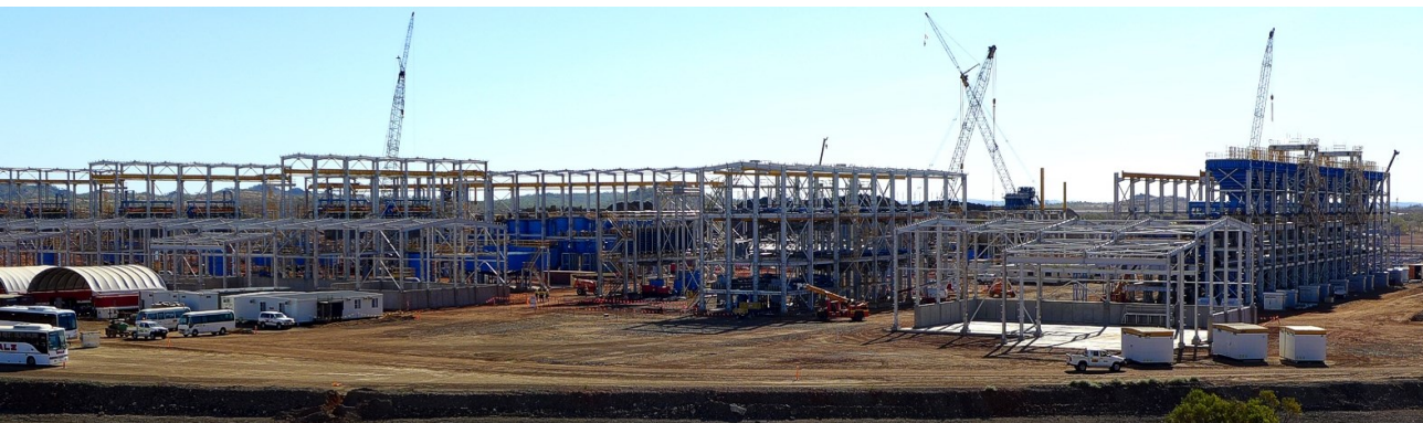
Figure 2: Rocklands Process Plant - major components installed, structural completion underway.
