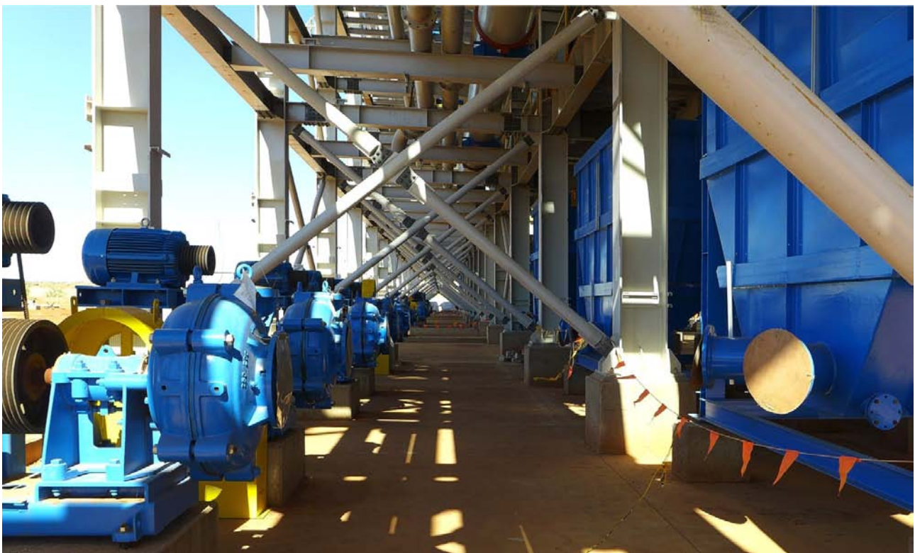
Figure 5: Gravity Jig building - light-fraction pump configuration
