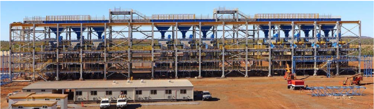
Figure 1: Rocklands Gravity Jig Circuit with multiple continuous gravity jigging units (alljigs®) supplied by German Company allmineral, capable of recovering various native copper fraction sizes (see flow-sheet diagrams from page 25)
