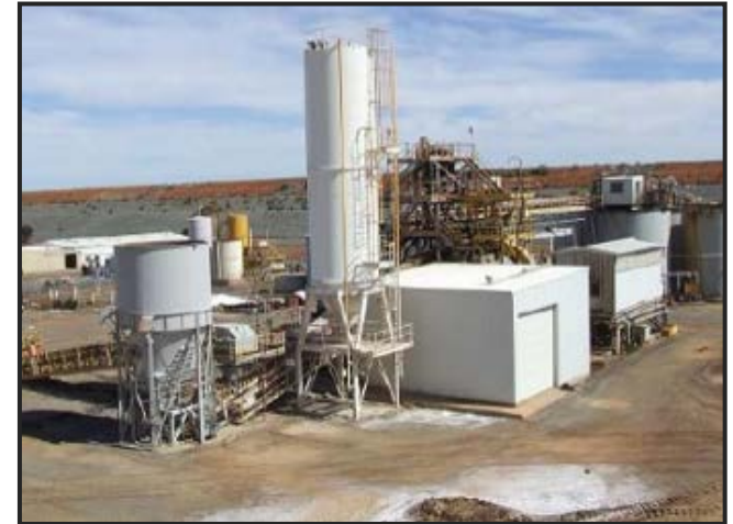
Kundana CIP Plant pre-decommissioning & refurbishment
