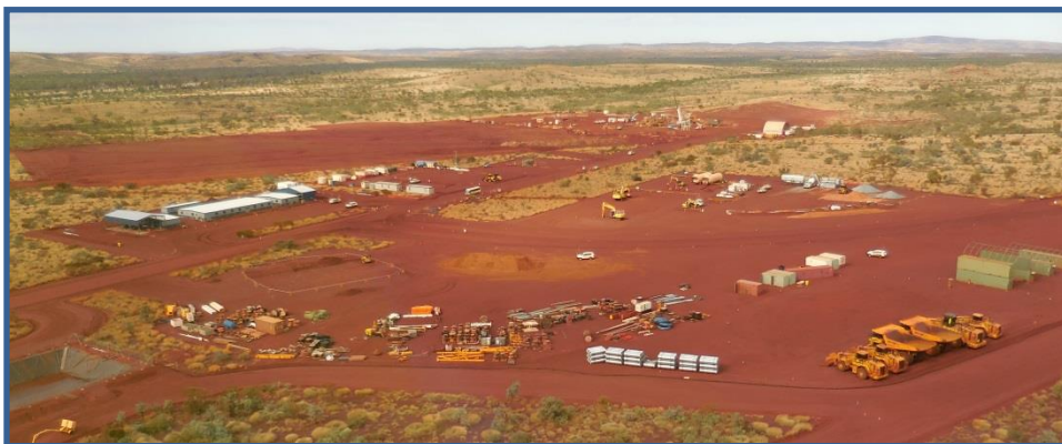
Iron Valley – Construction Underway (Image Date: 24 June 2014)
