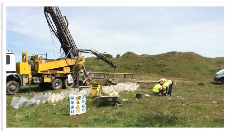
Figure 3: Drilling at Westside (Toro de Nueva Banco) in April. Waste from old mining visible as small mounds in the background.
