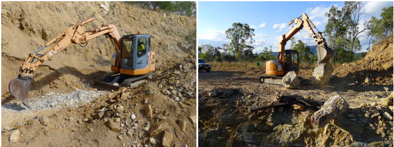
Figure 7: Excavating the bulk sample from the Frampton shear zone.
