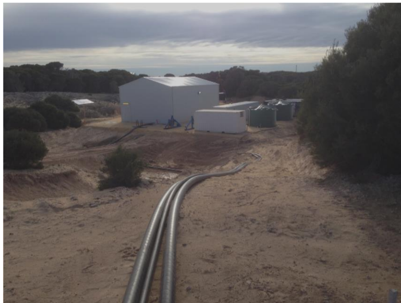
Perth Wave Energy Project pipelines connected to the power house and desalination plant, Garden Island, WA
