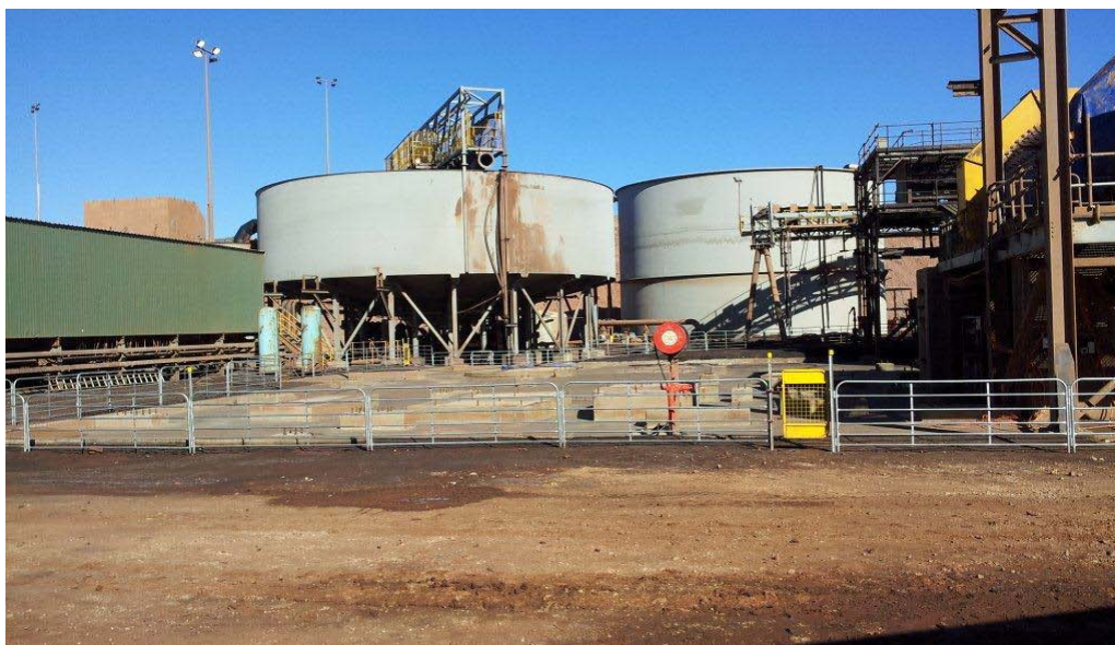
Photograph showing beneficiation plant site following completion of demolition
