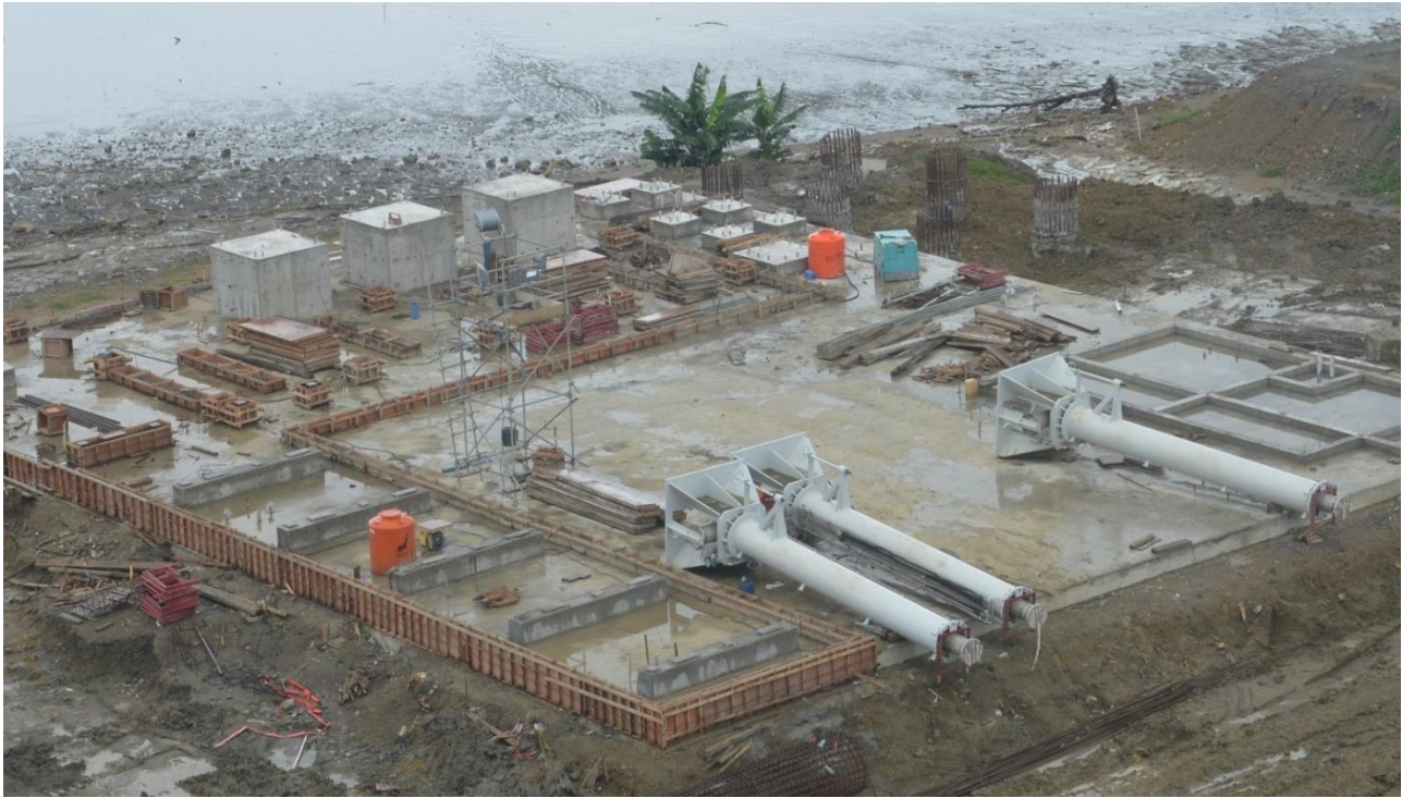
Construction of Jetty
