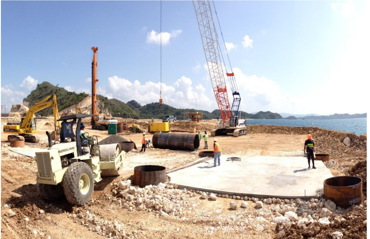
Construction of Jetty
