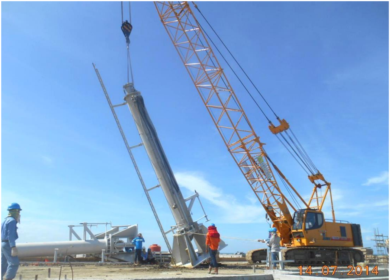
Erection of Marine Loading Arms
