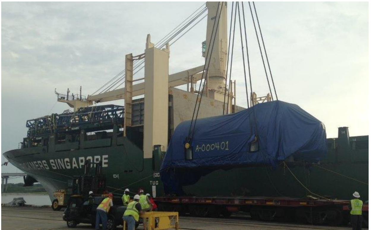
Loading of Turbine and Generator Unit 1 at Charleston Port in US
