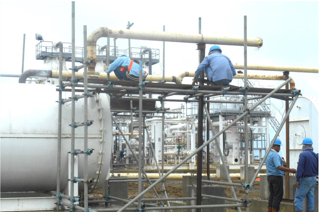
Fabrication & Installation of Interconnecting Pipe
