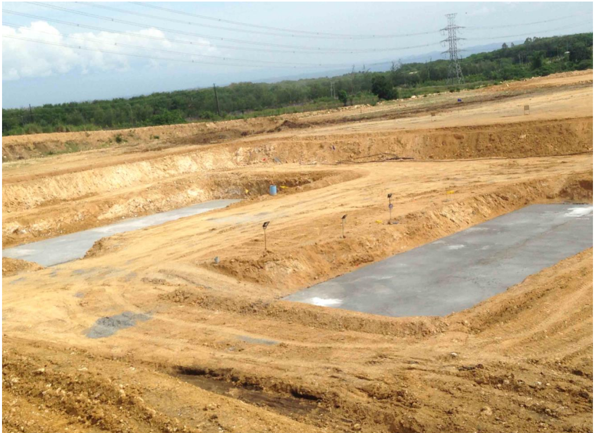
Site Formation of Power Station
