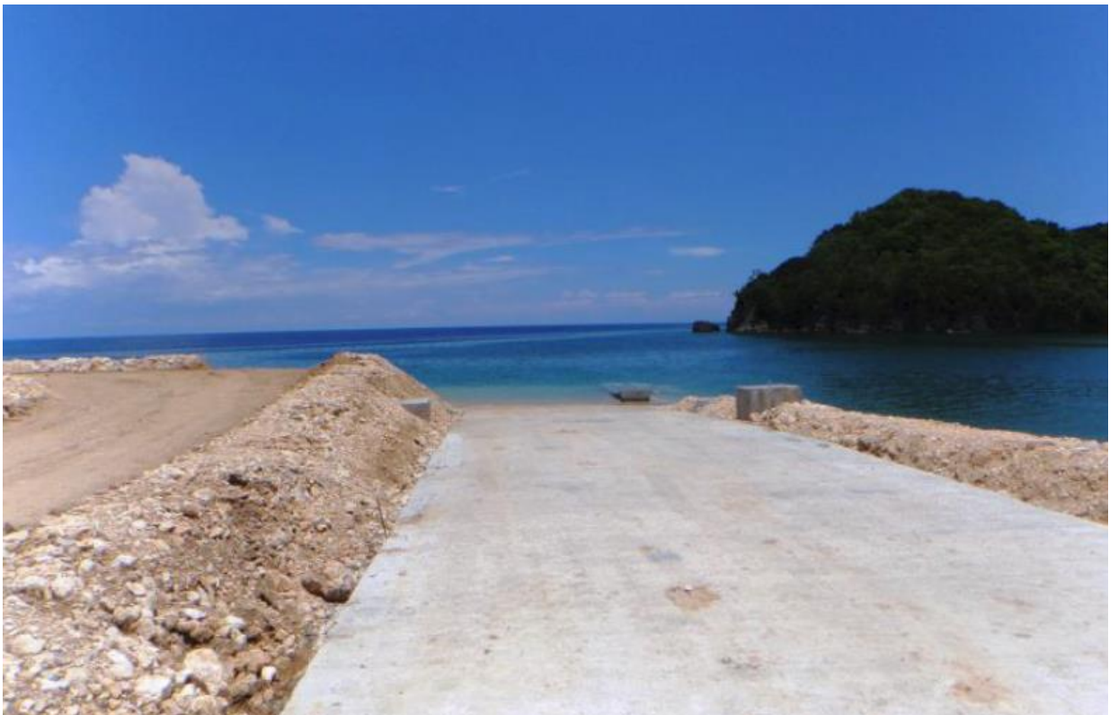
Construction of Heavy Loading Jetty
