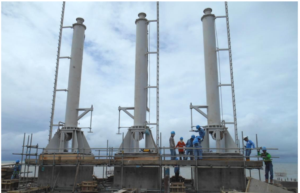
Erection of Marine Loading Arms
