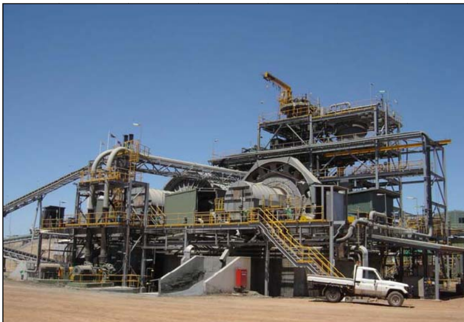
Figure 3: Black Swan grinding circuit
