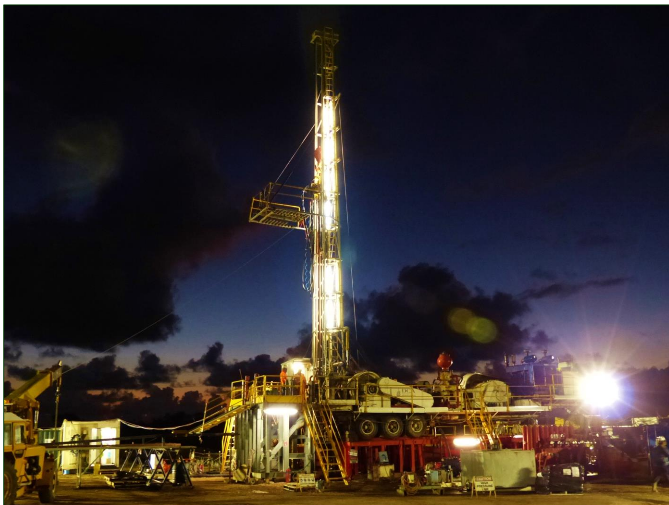
DCA Rig 7 night shift drilling ahead in the Kockatea Shale.
