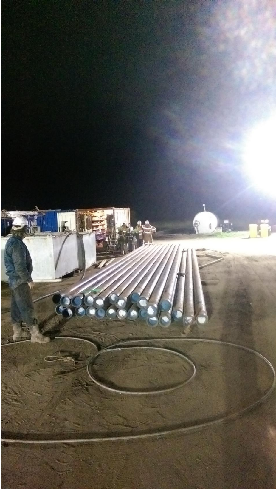
DCA crew preparing to run 7" casing
