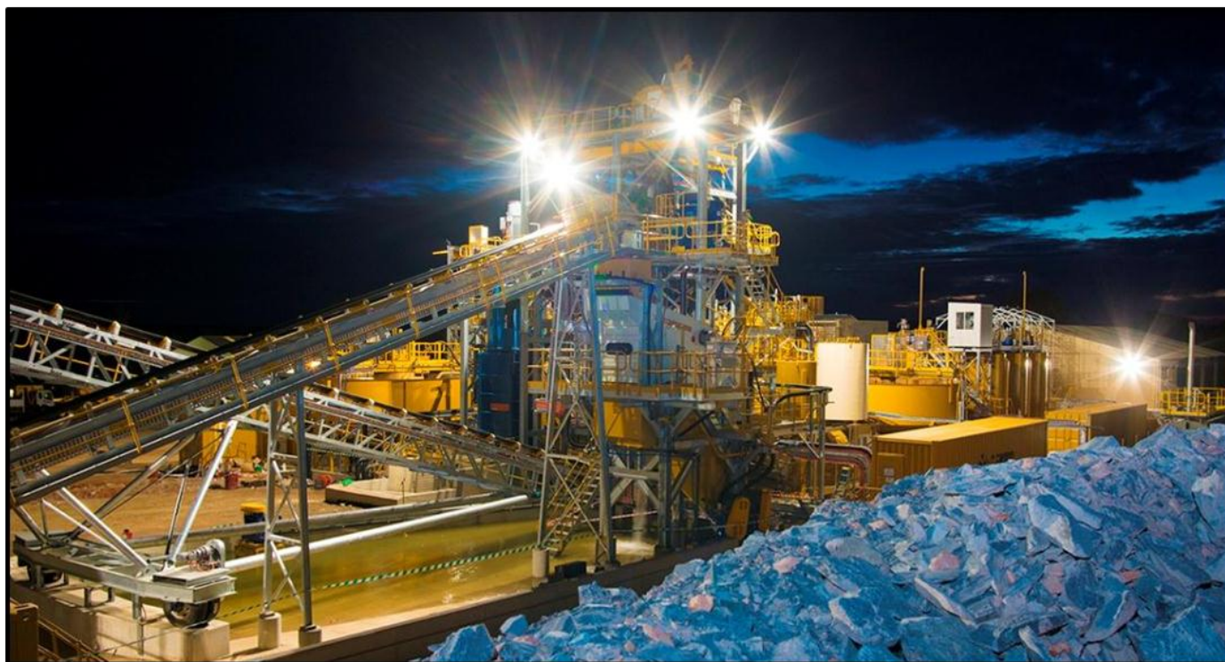
Hera Processing Plant
