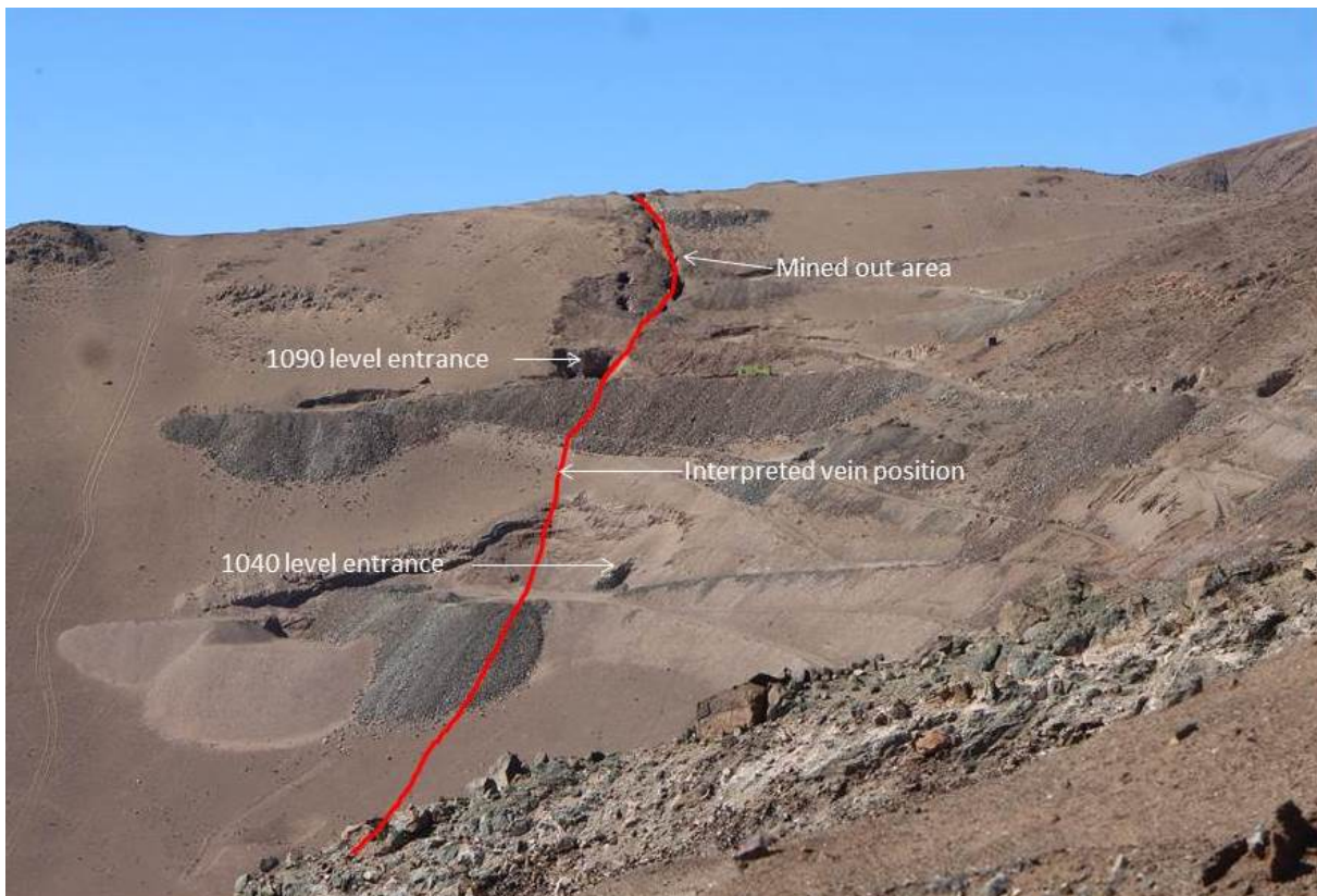
Figure 3 – San Sebastian mine and vein looking north. Note favorable topography for access, vertical distance between the 1040 level and 1090 level entrances is approximately 50m.
