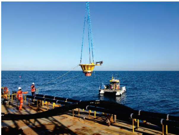
Installation of a Foundation Connector (left) and in place on an offshore foundation (right)
