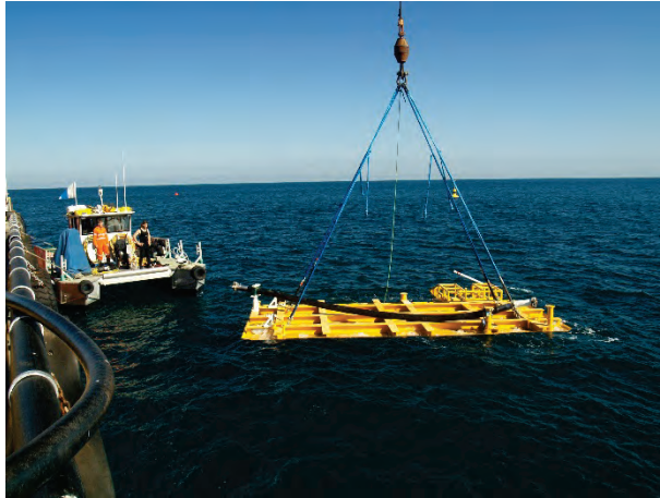
Installation of Pod mudmat (left) and Unit interconnection pipelines (right)
