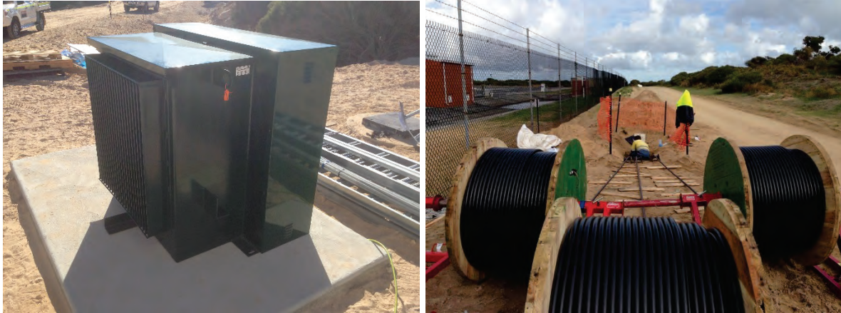
Onshore plant transformer (left), cable installation between the onshore plant and the grid connection point (right)
