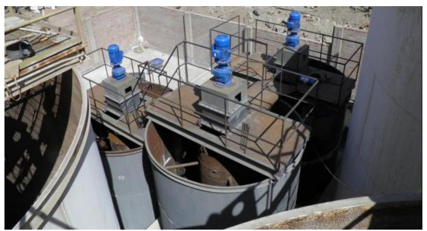
Picture 4: New carbon tanks installed prior to painting and wet commissioning.
