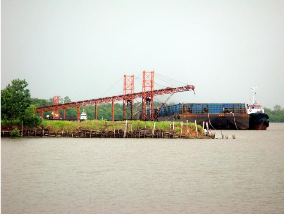
Figure 1: Coal loading facility at Batulicin *
