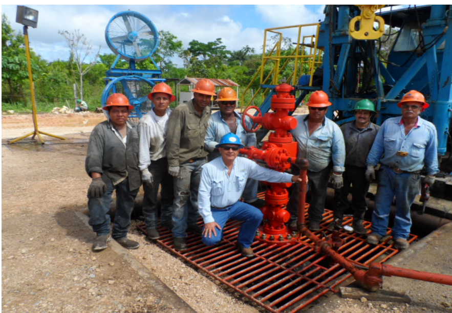
Atzam #4 Well Head- Commencement of Production, August 2013
